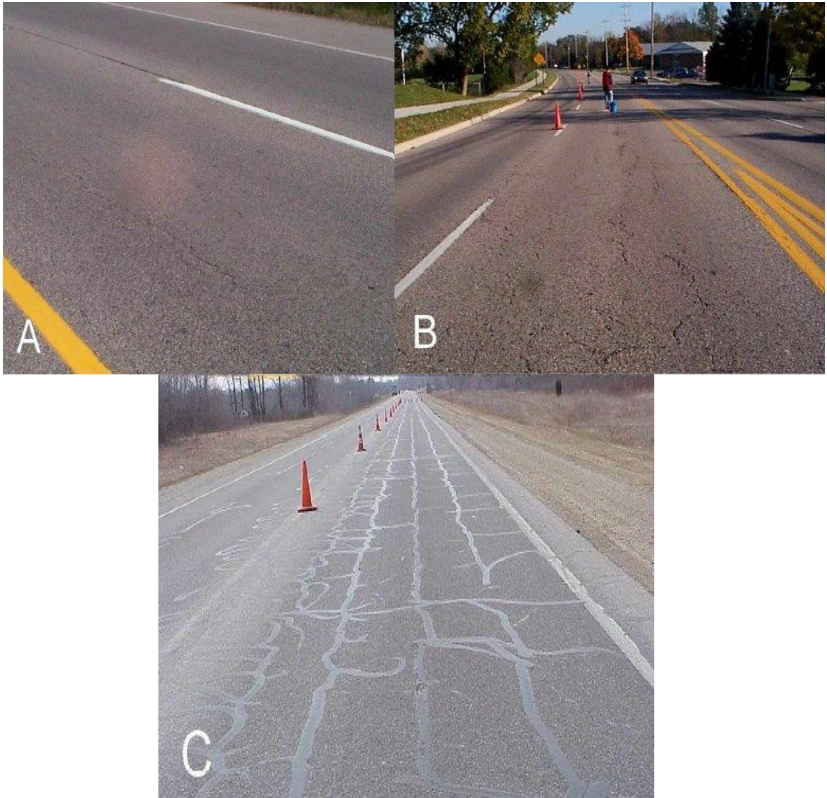
Figure 2-12 Photographs illustrating the development of top-down cracking (Svasdisant et al., 2002)
