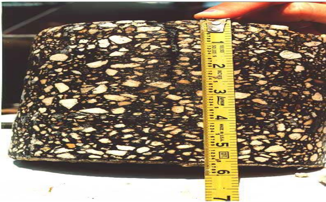
Figure 2-11 Core extracted from wheelpath shows top-down cracking (Myers et al., 2000)
